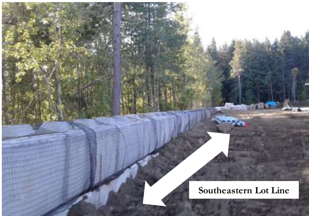
Figure 5: View of the Southeastern Lot Line Lock Blocks in Order to Have a Level Lot (Part of “Detail – C”)
